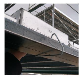
4. Push the plank upward to test whether the plank is securely fastened with the clip. Repeat the same steps on the other side of the plank.
