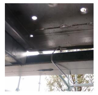
3. Ensure the end of the clip is hooked into the hole at the bottom of the plank.
